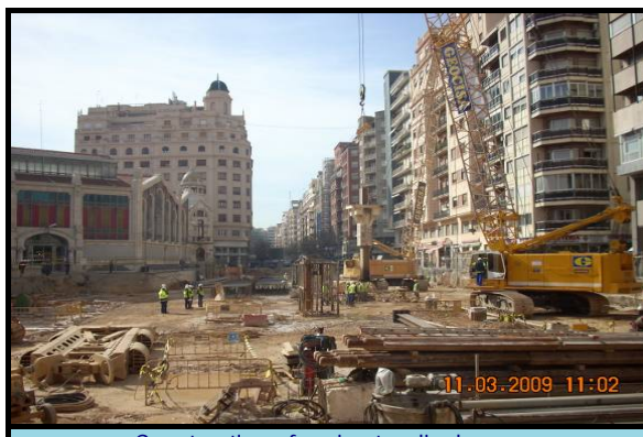
Construction of perimeter diaphragm
