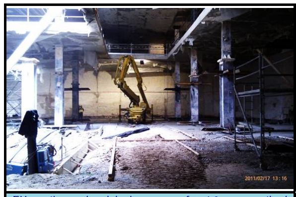
Excavation under slabs by means of "cut & over" method
